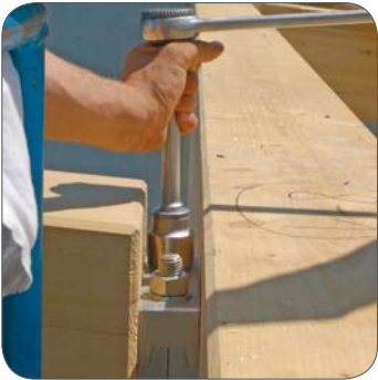
13:24 | Tighten the nuts.
