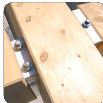
Connection finished: The secondary beams are placed in the clamping jaws.
