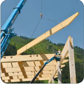
13:16 | After aligning the secondary beam, MEGANT® is hooked.
