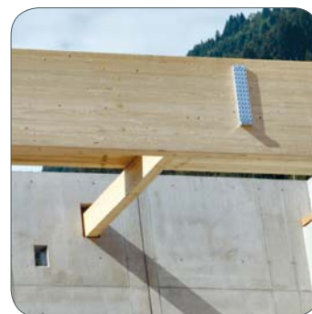
With only 2 cm hooking way, a mounting in cutouts of concrete walls can be done.
