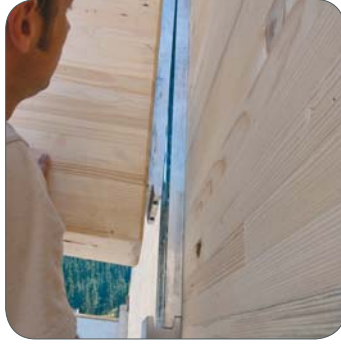
13:21 | For threading and dropping, MEGANT® requires only 2 cm.
