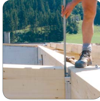
13:23 | Insert the threaded rods and drill them into the caps.
