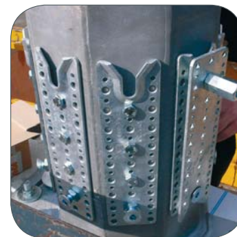
First node for dome
