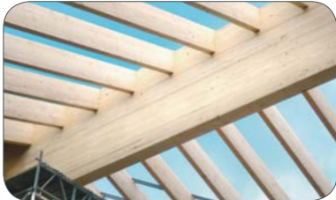
Hall roof of carpentry S. Hinrichsen (Germany)
