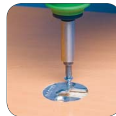
3) Screwing with CS-screws
