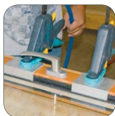
2) Pressing pane of glass against outer seal
