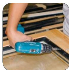
3) Screwing or nailing the FIXclip-Profile
