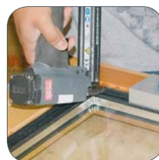
3) Screwing or nailing the FIXclip-Profile
