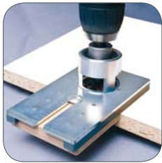
1) Drilling with jig
