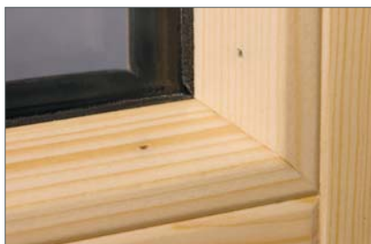
Conventionally glass bar attached with exposed nails
