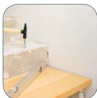
2) Gluing and install
