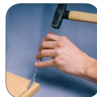
4) Knock in with the insert tool
