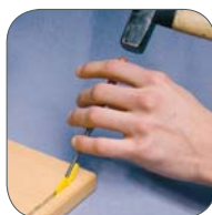
3) Knock in with the insert tool
