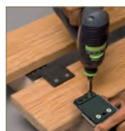
Fasten to the boards with screws
