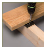
Fasten to the joists with screws
