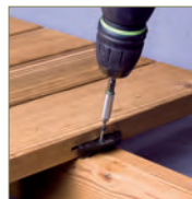
Fastening with screws
